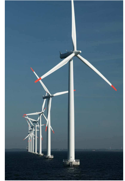
Offshore wind farm
